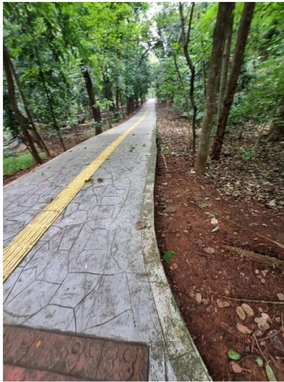
Picture 5. No street lighting.
