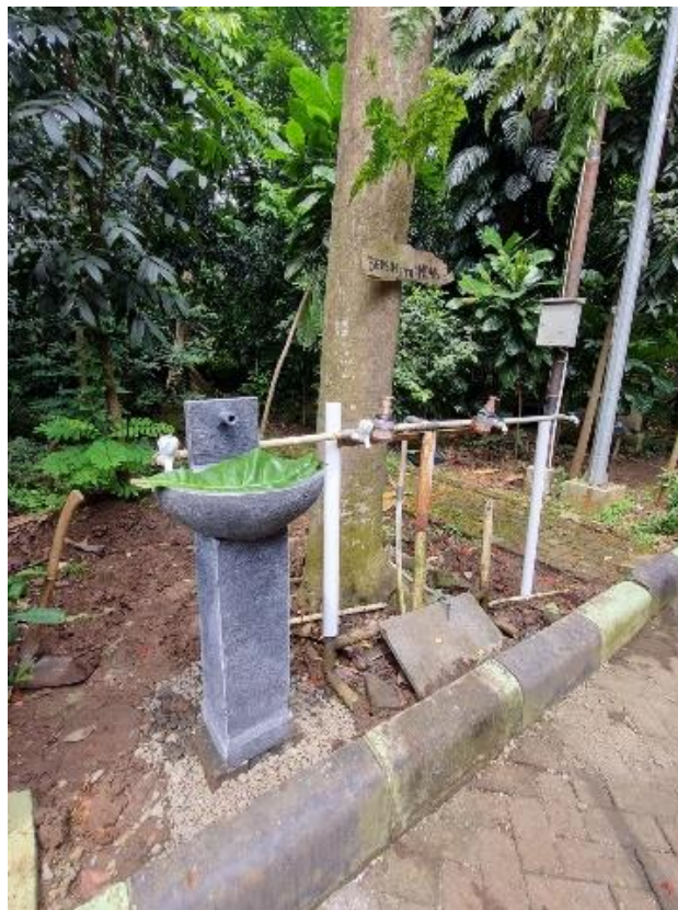
Picture 3. Existing Facilities
