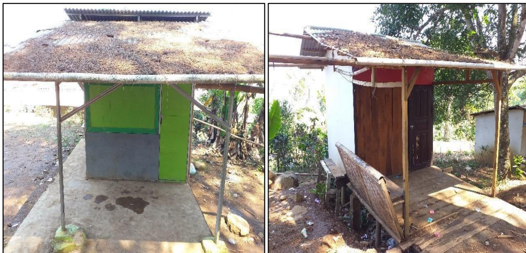
Figure 2. Stall Condition During Location Survey
