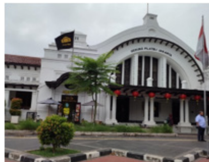
Figure 1 Facade of Pos Bloc of Adaptive Reuse Gedung Filateli, Jakarta (Source: private collection, 2023)
