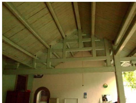
Figure 8 The Supporting Structure of the Roof (Source: Researcher Team, 2013)
