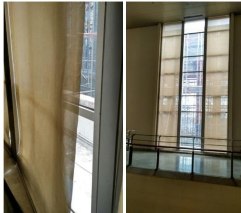
Figure 2 The Use of Curtain as Treatment to Lessen the Glare Effect, The National Museum (Source: Wulandari et al. , 2016)
