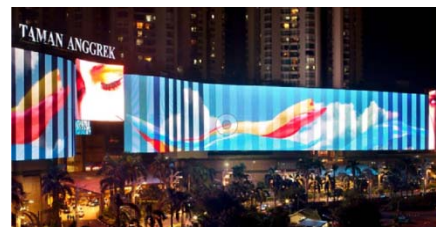
Figure 6 Screen Giant LED Façade Mall Taman Anggrek at Night (Source: www.lighttalk.via-verlag.com )
