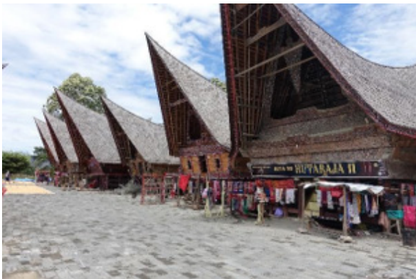
Figure 8 Physical Aspect in Ulos Hutaraja Village: Product Displays in Local’s Traditional Houses (Source: Private Document)
