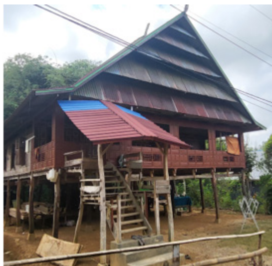
Figure 9 House in Outer Kajang (Author, 2023)
