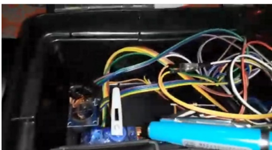
Figure 5. Safe Deposit Box Installation In Inside View
